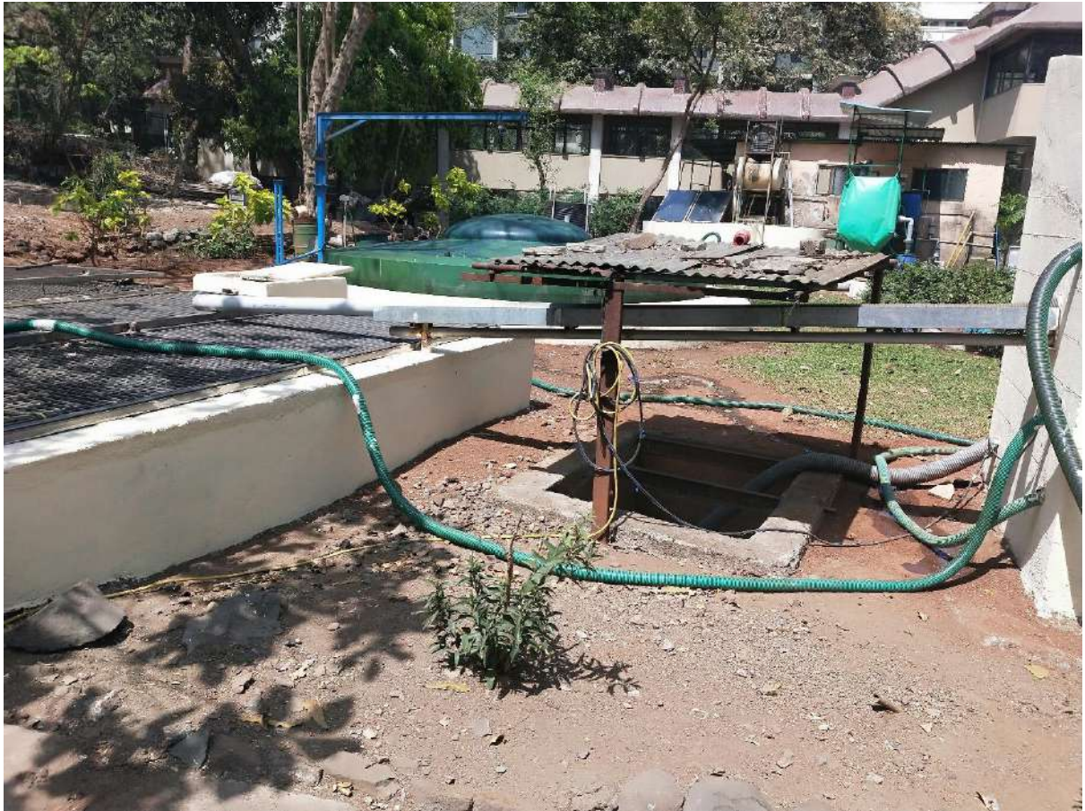
Biogas plant at BARC-Anushaktinagar
