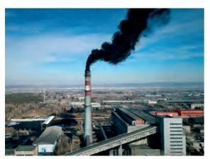
Fig. 2(a): A typical coal fired thermal power station. A typical 500 MWe coal fired unit releases about 10000 tonnes per day of CO2, which has major bearing on green-house effect. In addition, copious amount of So<sub>2</sub>, NOX gases and harmful Particulate Matter (PM) amonust others are also released. In the year 2021 India emitted about 1.4 billion tonnes of CO, owing to coal firing at power stations alone
