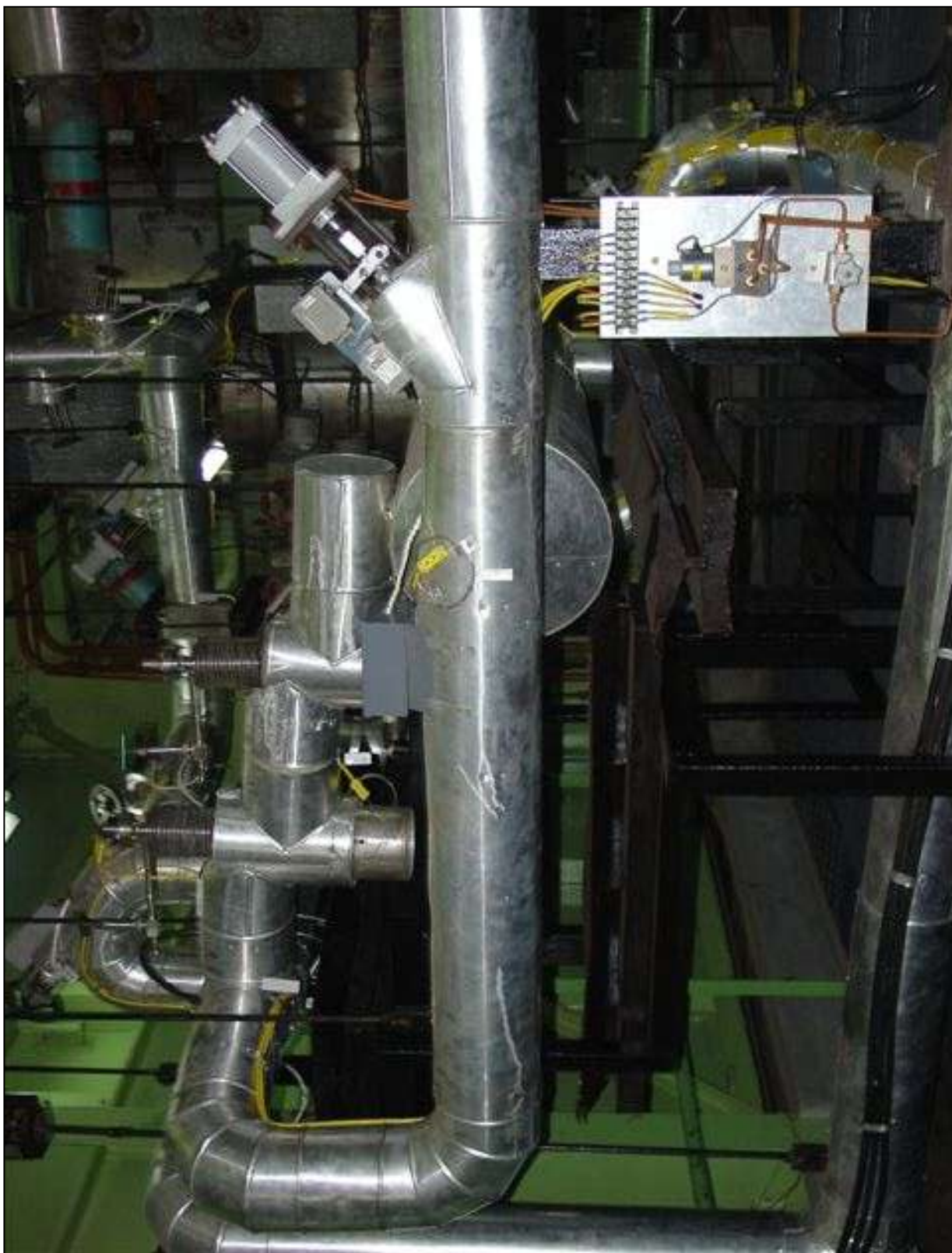
Fig. 3.17: Triplicated systems of SG leak detection photo
