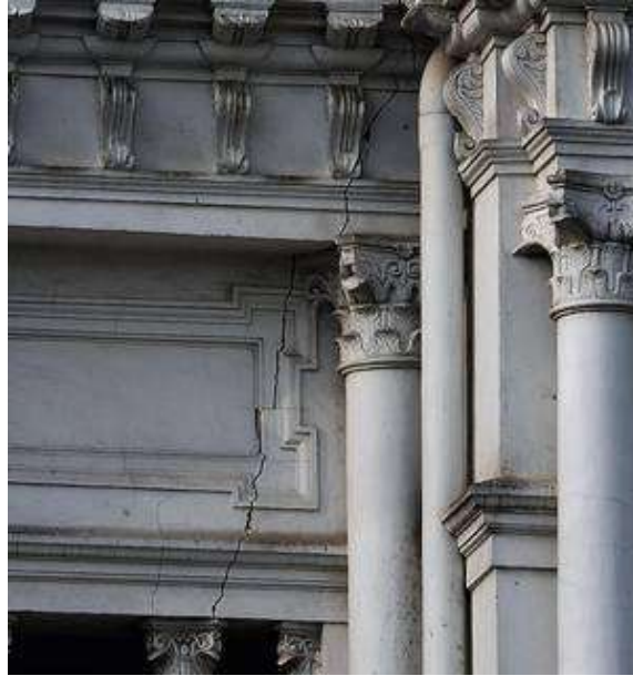
Fig 1. 4: Cracks in Rippon building due to excavation for Chennai Metro Rail construction
