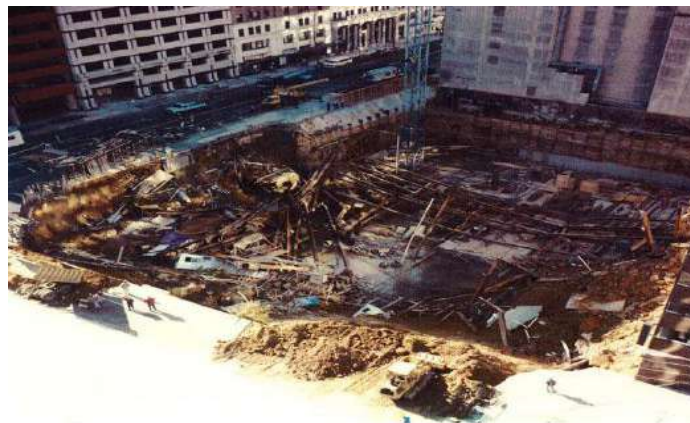
Fig 1.2: Failure of an open excavation Washington DC
