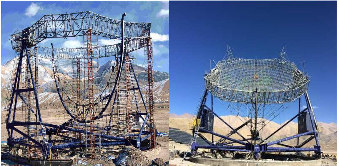
Figure 4.17: The left panel shows the installation of MACE 21m diameter dish at Hanle in November 2015. The right panel shows it on October 16, 2016
