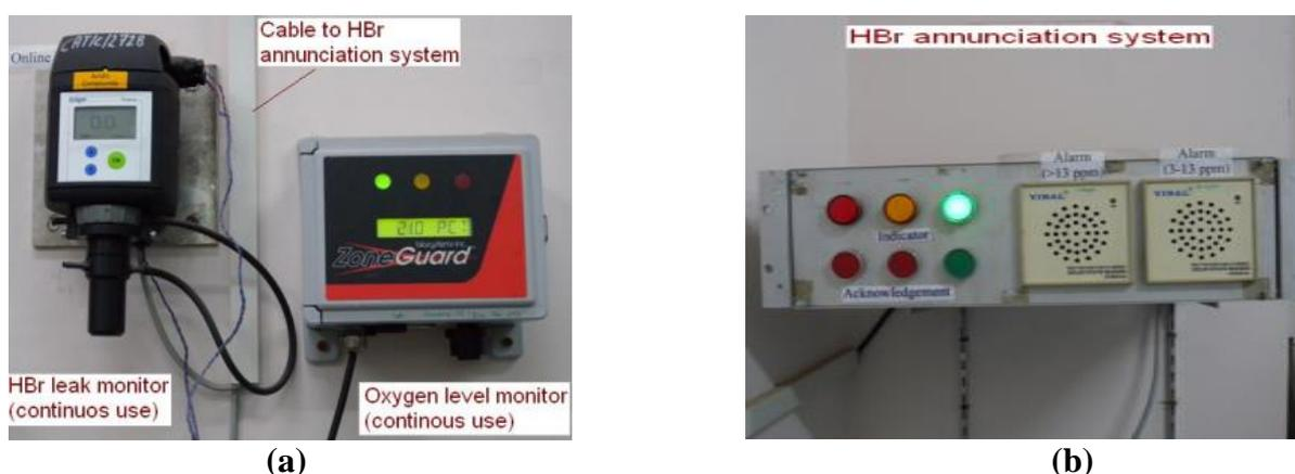
Fig. 2.7 Photographs of installed HBr sensor, oxygen monitor(a) & HBr alarm system (b)
