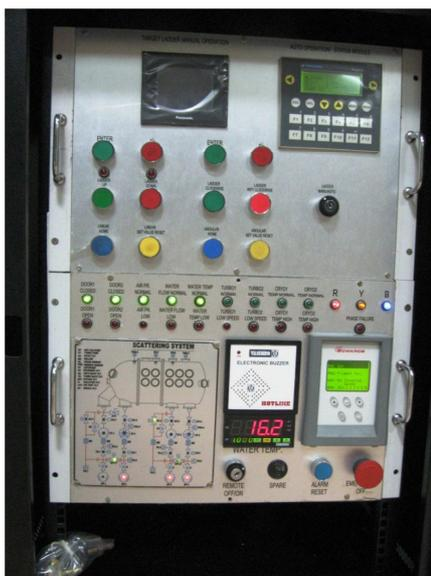
**Figure 6.9:** Remote control panel of target ladder. It also shows the status all operation of target ladder and pumping system.
